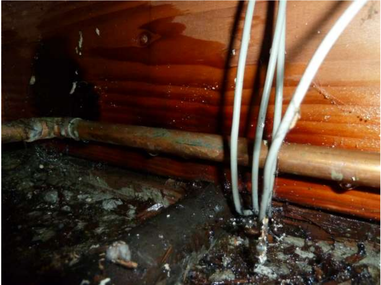
This is the same picture you can see the small mist of water against the wood just above the pipe.
